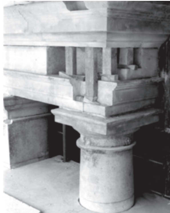
Repairs in progress to the entablature on the south side of the east window.
